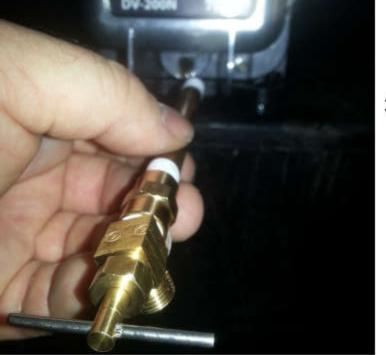
4. Tighten drain with a 7/16" wrench (Snug do not over tighten)
